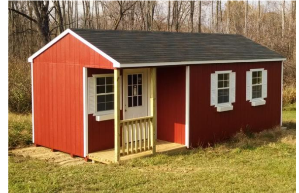
36" 9-Lite Steel Door, 3/4" T&G DryPly Floor, 3 24x36 Windows, and 4' porch
